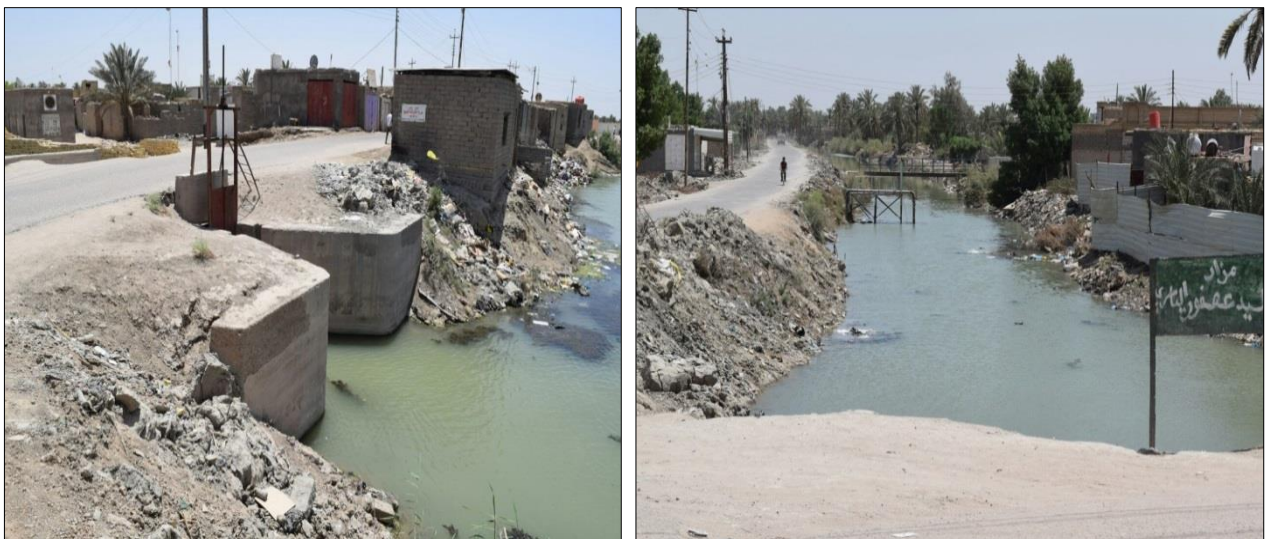
Figure 20. Photos for Al-Kurmashia regulator and canal, taken by Samir Najeeb Makki, May 2017.
